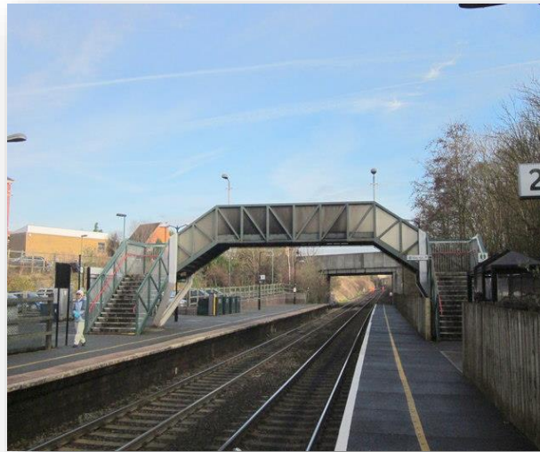
Bromsgrove station in 2015 prior to rebuilding
